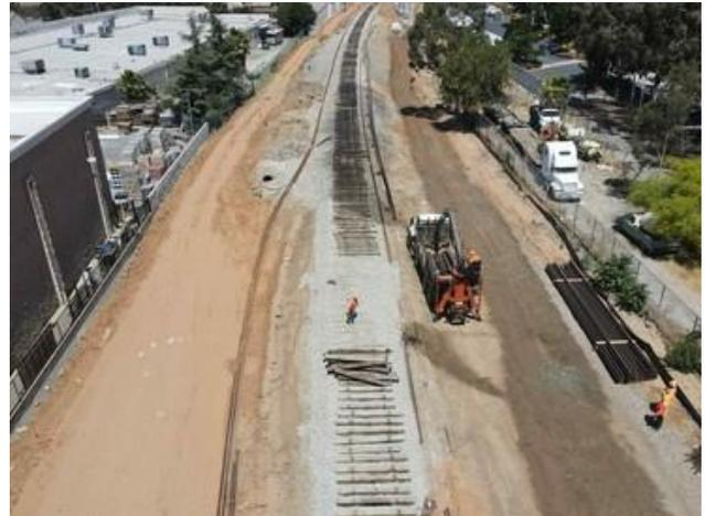
As seen in the photo above right, crews have now begun removing the old freight track through the city of San Dimas as part of the next segment of freight track relocation. In all, three track shifts are anticipated to take place in 2021, allowing crews to fully focus on installation of the light rail system starting next year.
